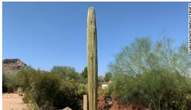
A 4G and 5G capable cactus in the Scottsdale, Arizona area built by Valmont Industries
