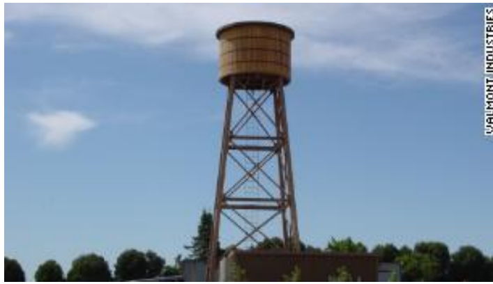
A faux-water tank conceals 4G equipment in Schellville, California. It can be modified to be 5G capable.
